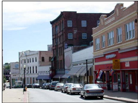
Figure 3. View looking east on Main Street.
